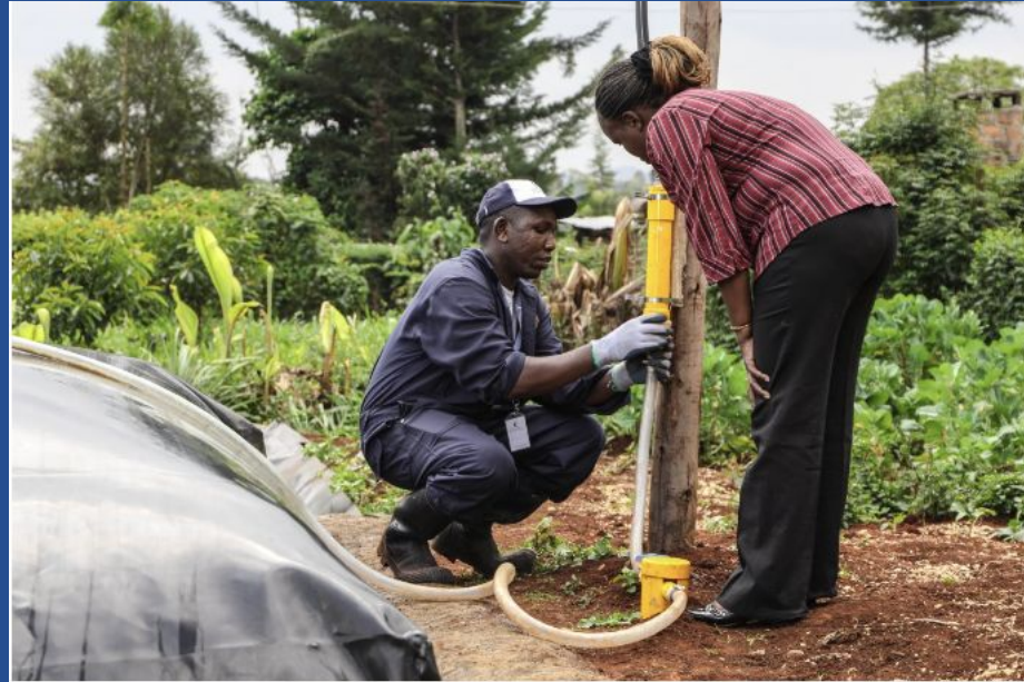
A biodigester is installed in a community in Kenya. (Photo: Sistema.bio)
